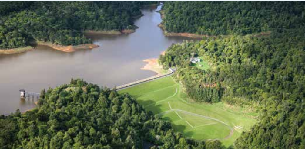
Cosseys Dam in the Hunua Ranges "will take a lot of beating as a site," says Wal.
